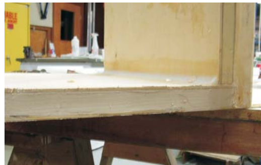
Epoxy/410 Microlight is used to fill and finish the edges.
