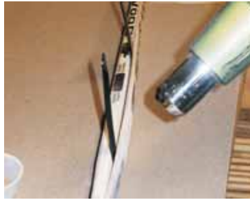
1. Open the split, clean out any loose material, and warm the area with a heat gun.
