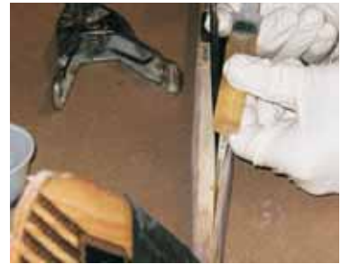
2. Inject G/flex 650 into the split. Work the mixture into the crack.
