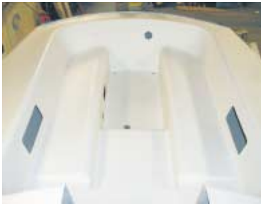
The cockpit after priming with US Paint™ epoxy primer white base, applied with an 800 foam roller.
